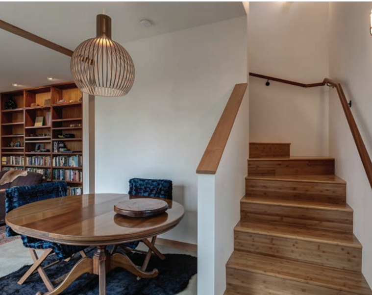
Intentional spaces and living. The winder staircase is one of the most efficient of designs.
