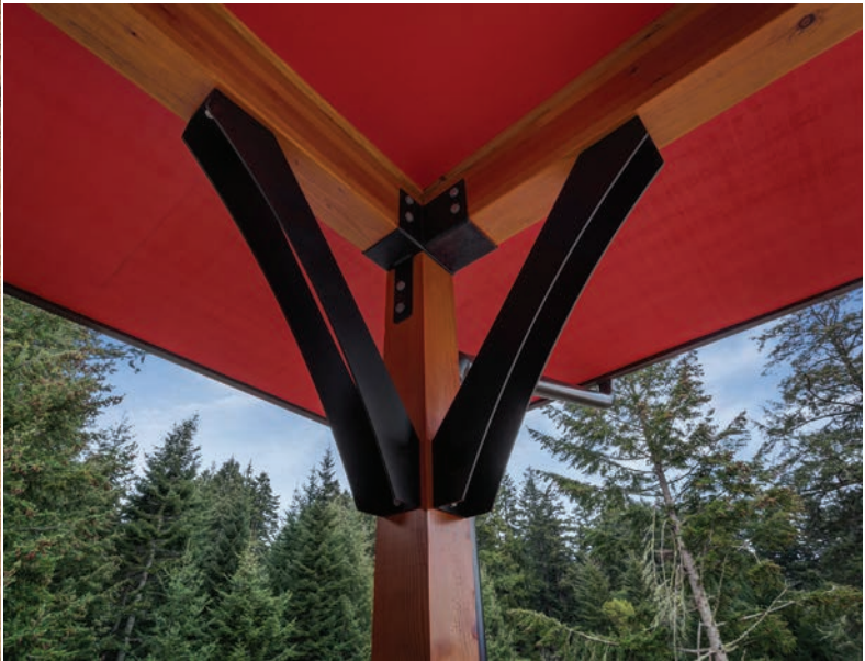
The gentle curve and proportions were derived by using the golden mean - an age old architectural trick. It ensured the brace proportions related to the overall structure.
